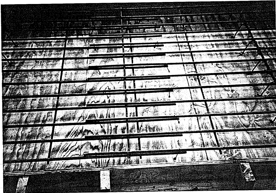
Figure 3.13: Photograph of Lap Splice for Slab UD20-1
