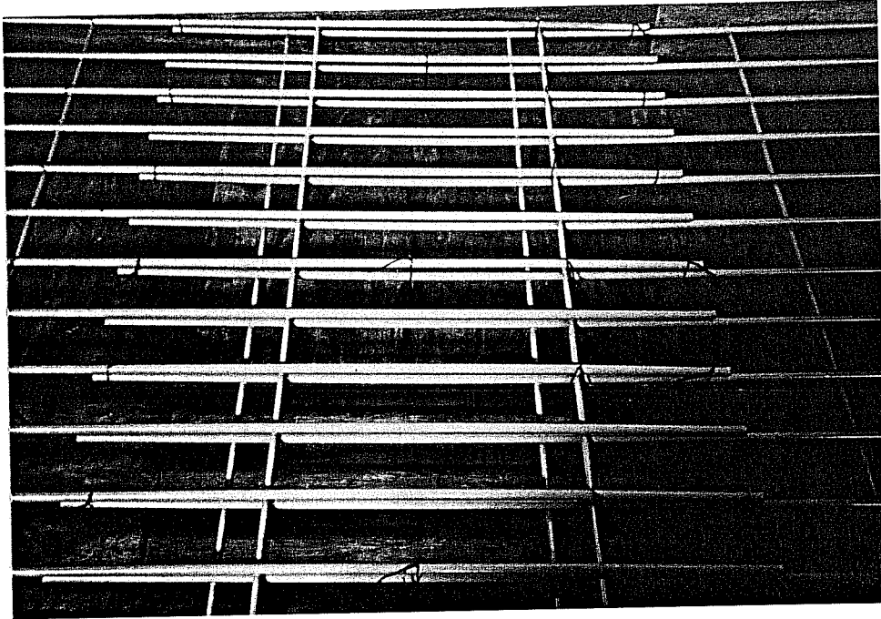
Figure 3.12: Photograph of Lap Splice for Slab CW20-1
